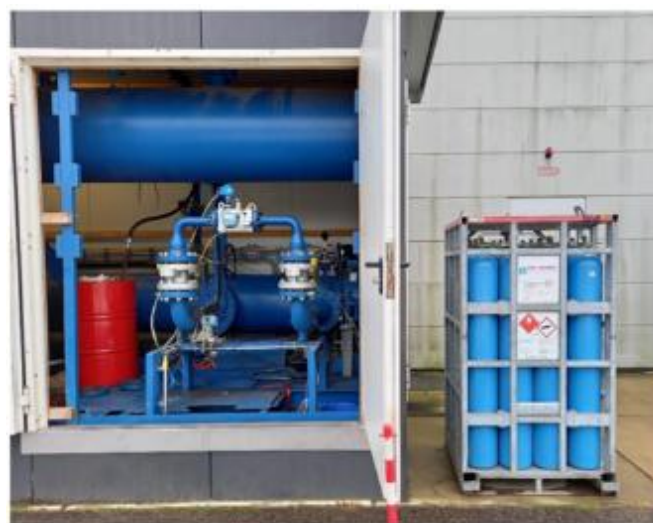
Figure 1. MuT mounted on VSL's GOPP, accompanied by hydrogen gas cylinders.
